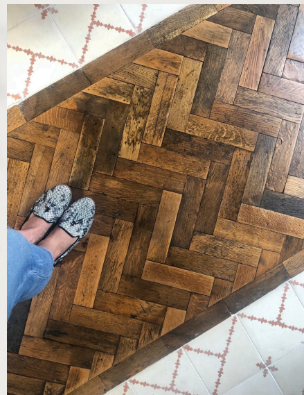
Refurbished parquet flooring
