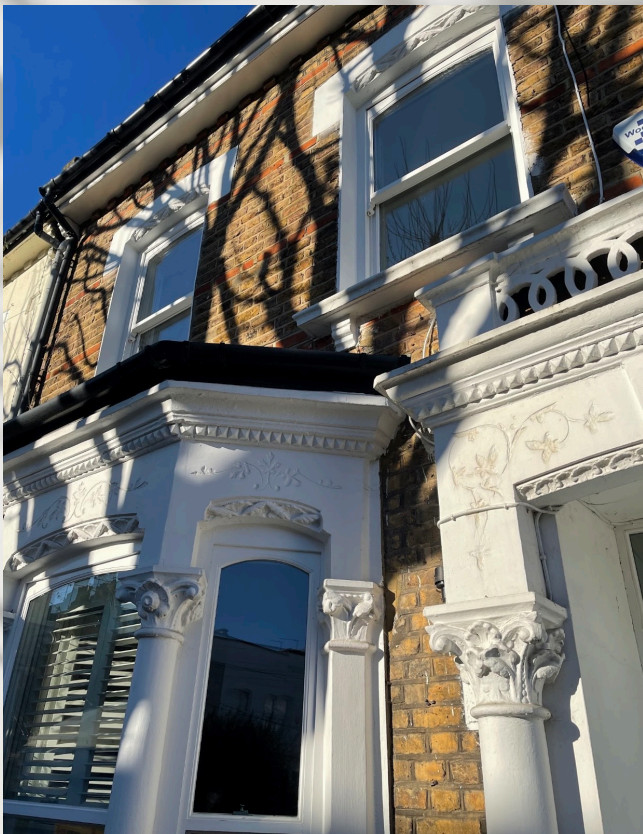
Finsbury Park project
